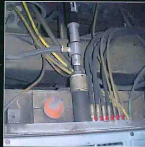
Foundry application: VDF pump solves maintenance problem
